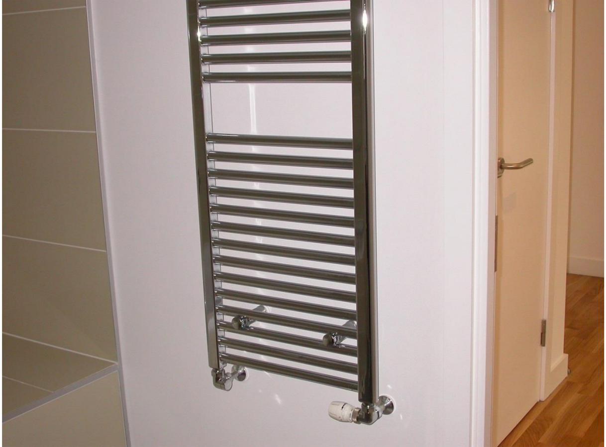
These will ONLY operate when the underfloor heating is switched on. The control can be adjusted to regulate the amount of hot water flowing through the rail from 0 (off) to 5 (max).
