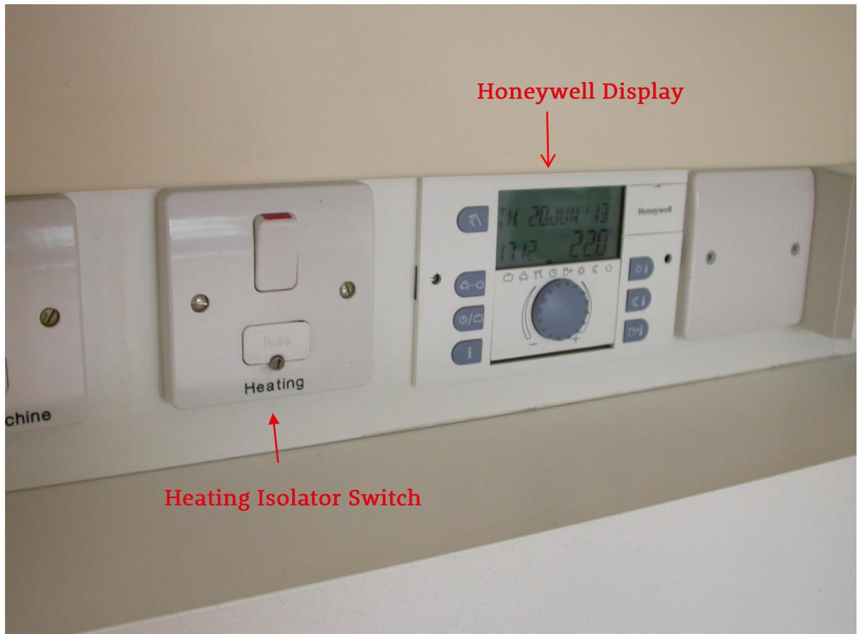
The **Heating Isolator Switch** (image above) turns the hot water and heating supplied to your home on and off. **We recommend that you do not switch this off as it can affect the settings to your home and could have cost implications in addition to health and safety issues.**
